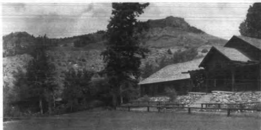
A CORNER OF A RANCH HOUSE
