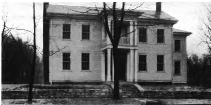
Holt House, January 1, 1941. Note: This shows the exterior complete except for green window shutters
