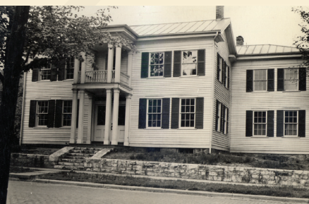
With the renovation complete, Holt House was officially reopened on April 26, 1941.
